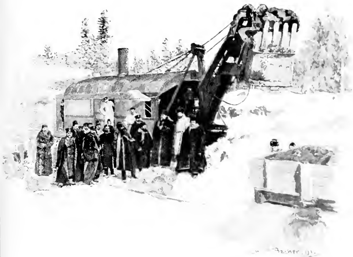
An American Steam Shovel at Work on the Moscow, Jaroslav & Archangelsk Railway between Vologda and Archangelsk, Russia.
